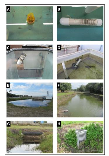
**Figure 3.** Examples of physical barriers used at a tropical fish farm. Similar physical barriers may be used at other types of aquaculture facilities, scaled to appropriate sizes. Barriers include screens on tanks vats (A, B, C, and D), detention pond (E; water is eventually discharged), retention pond (F; water is not discharged), and riser board control structures (G and H).
